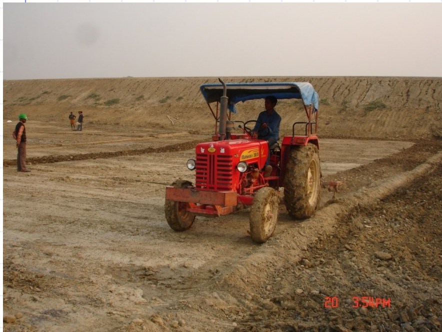
◇ Relaying of top soil
