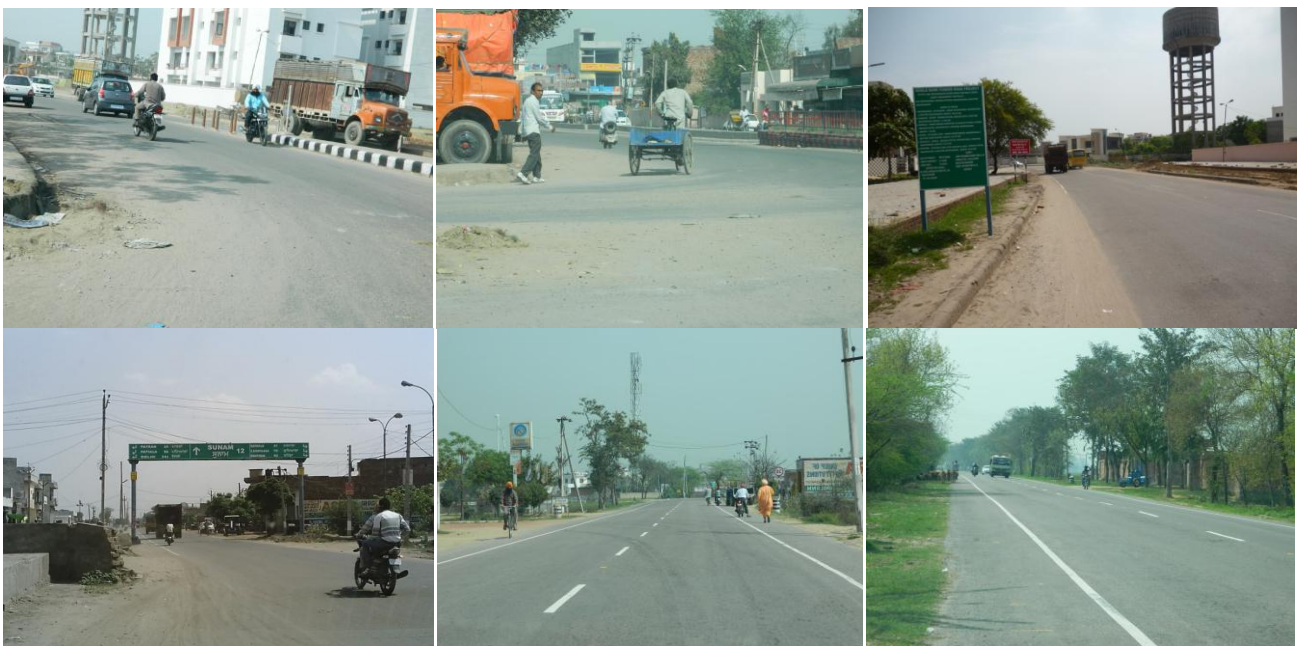
Figure 2-1: Photographs of Project Road
