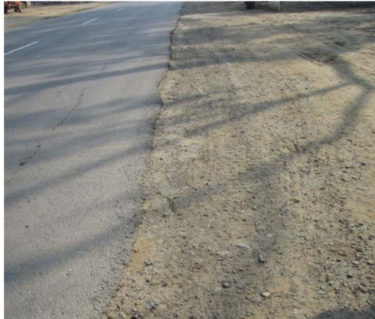
2. Low Level Pavement Shoulder: S2 - (34+100 L.H.S)
