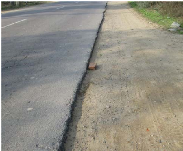
3. Low Level Pavement Shoulder: S - 2 (40+900 R.H.S).
