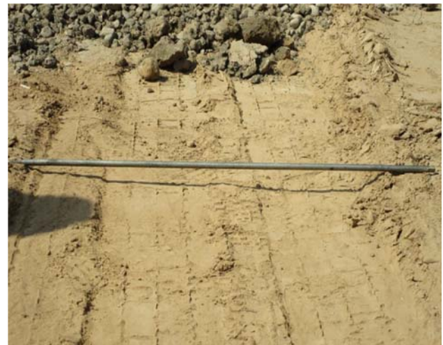
7. Improvement work in progress: S4 - (17+500 R.H.S)
