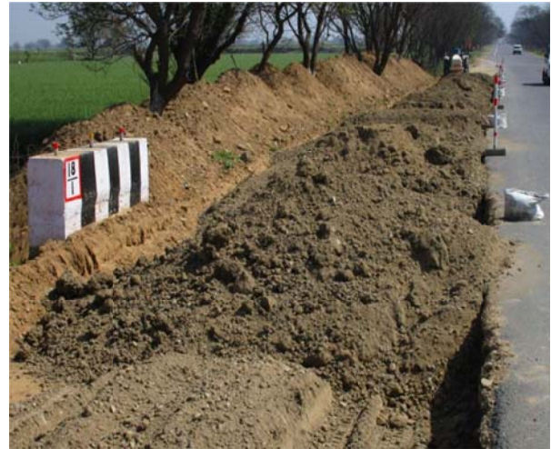
10. Crushed material used for GSB: S4 - (17+550 R.H.S)
