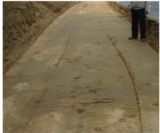
5. Improvement work in progress: S4 - (21+420 L.H.S)
