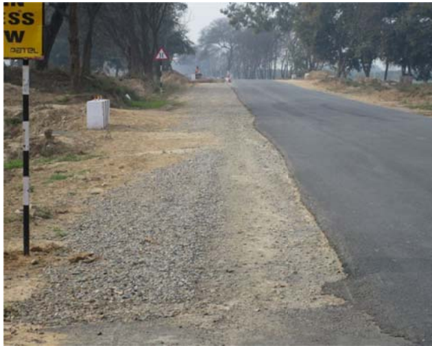
4. Improvement work in progress: S4 - (21+400 to 21+500 L.H.S)
