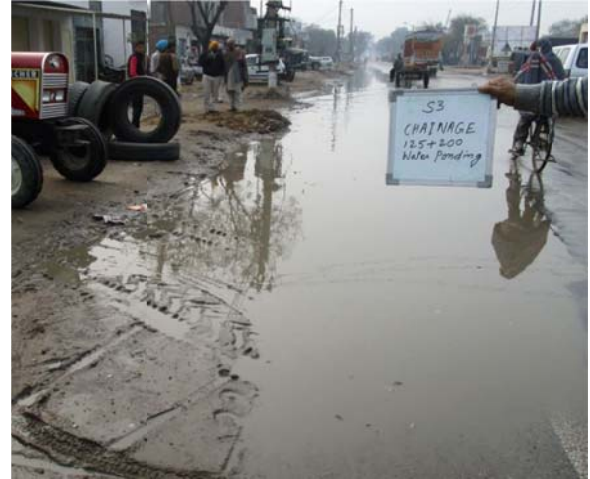
2. Drainage water adjoining pavement edge: S3 - (6+200 R.H.S)
