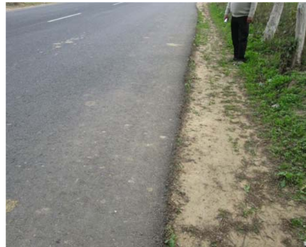
2. Unsealed earthen shoulder B8 - (24+140 R.H.S)
