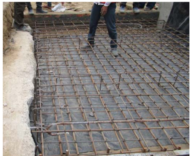
4. Bottom Main Bars (work in progress) S - 2 (45+100 R.H.S)
