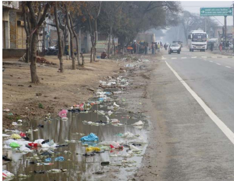
8. Water Stagnant: S4 - (15+150 R .H.S)
