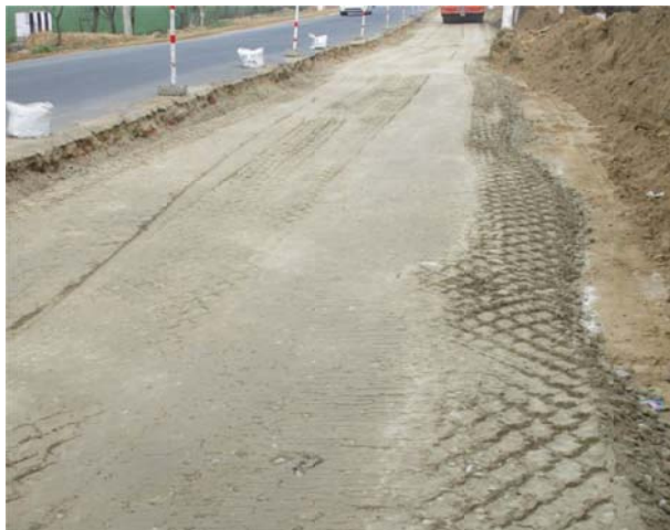
2. Preparing GSB (work in progress): S4 - (16+680 L.H.S)
