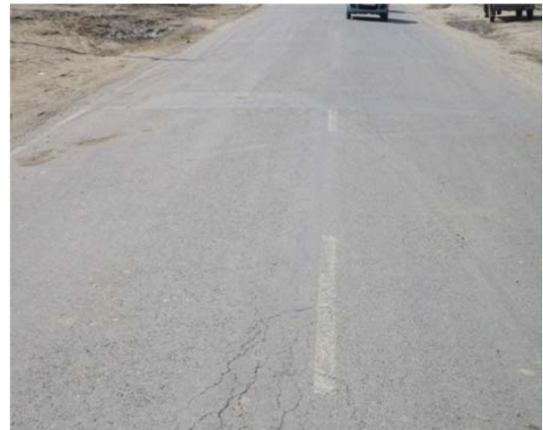
4. Worn out pavement marking: S3 - (124+820 Centre)
