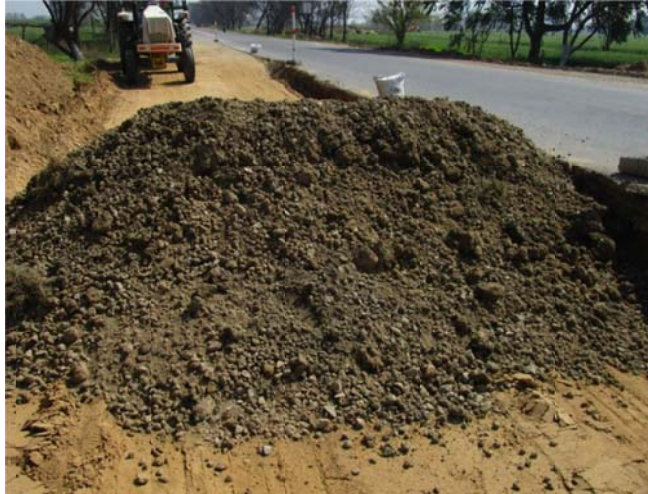
9. Crushed material used for GSB: S4 - (17+510 R.H.S)
