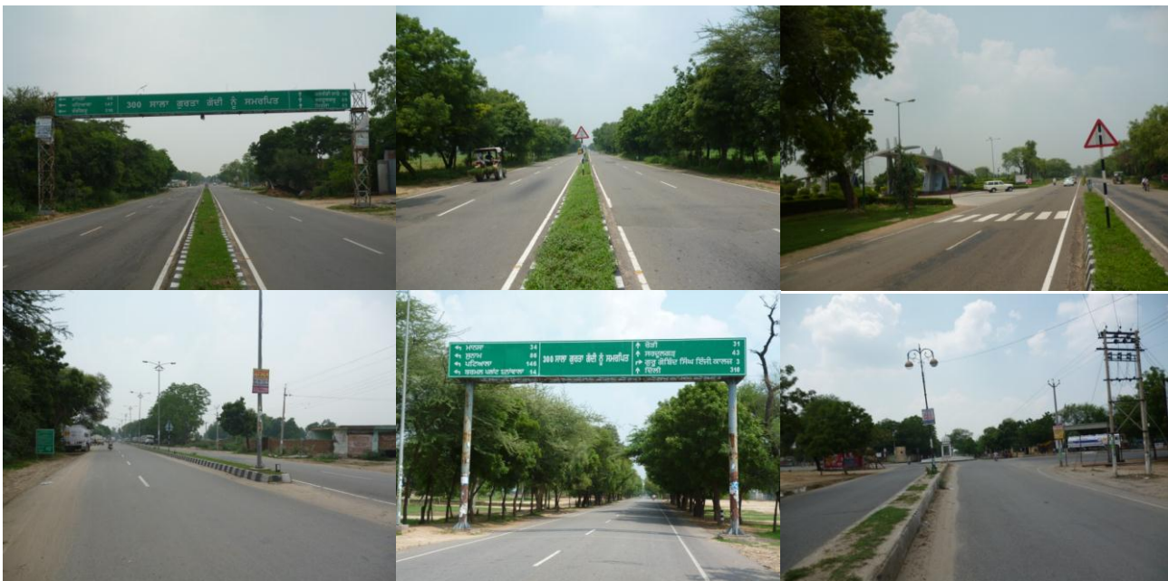
Figure 2-1: Photographs of Project Road
