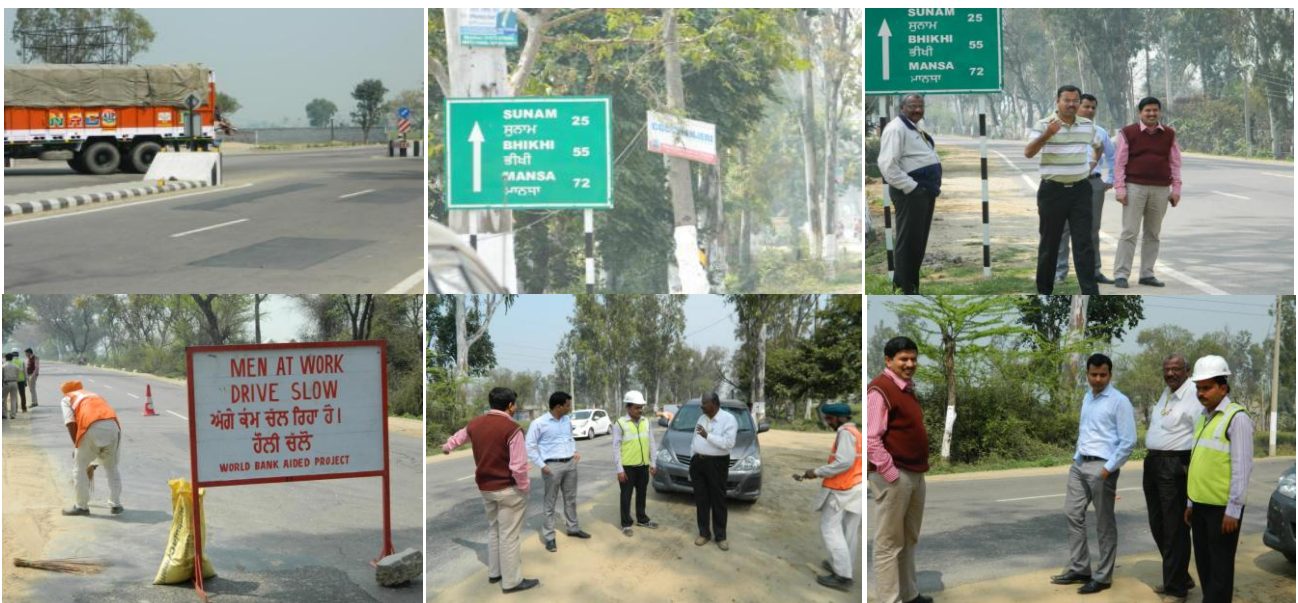
Figure 2-1: Photographs of Project Road
