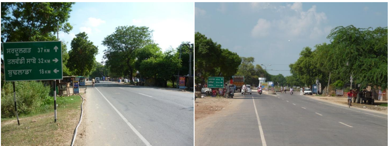
Figure 2-1: Photographs of Project Road
