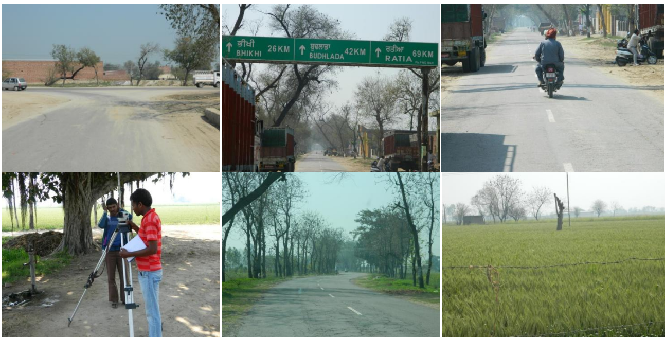
Figure 2-1: Photographs of Project Road
