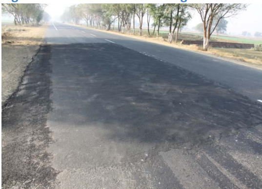
Figure 1-4 : Sector S4 – Patching km 14+000
